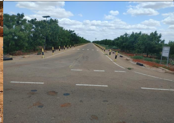
Greening at New County Headquarters
