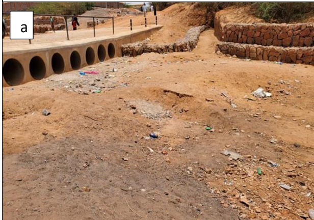
Storm water protection works
